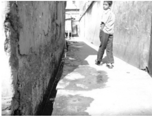
Fig. 4: Open drain with low capacity
