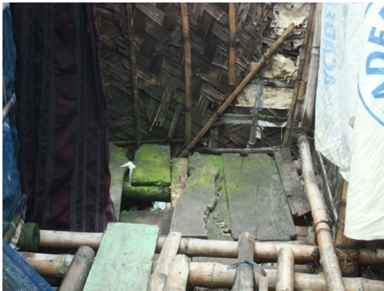
Figure 4: latrine facility; Source: Field Survey, 2011
