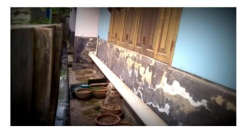
Figure 2: Use of setback as open drain Source: Field Survey, 2015.
