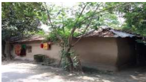
Source: Field Survey, 2016. Figure 3. Kutcha House.
