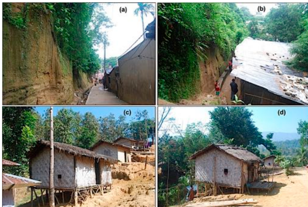
Figure 19. (a,b) Systematic hill cutting in the Lalkhan Bazaar area in CCC, and (c,d) a typical tribal housing in the Sandak Para community (21°48′37.17″N and 92°26′13.55″E), Thanchi, Bandarban, Bangladesh. Source: Fieldwork, 2014–2016.
