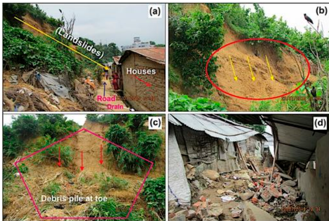
Figure 1. Landslides in the Lalkhan Bazaar area, Chittagong City Corporation (CCC), Bangladesh. (a) Location of vulnerable houses; (b) landslide scar; (c) landslide deposit; and (d) destroyed houses. Source: Fieldwork, July 2015.
