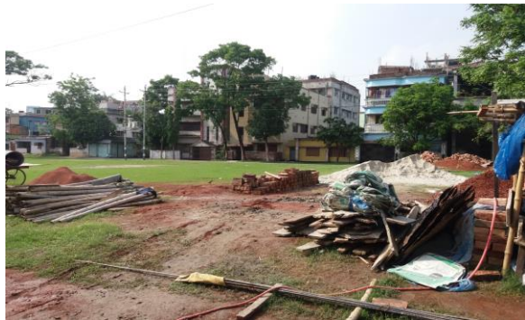
Fig. 7: Construction debris in Uposhohor open space, Rajshahi.
