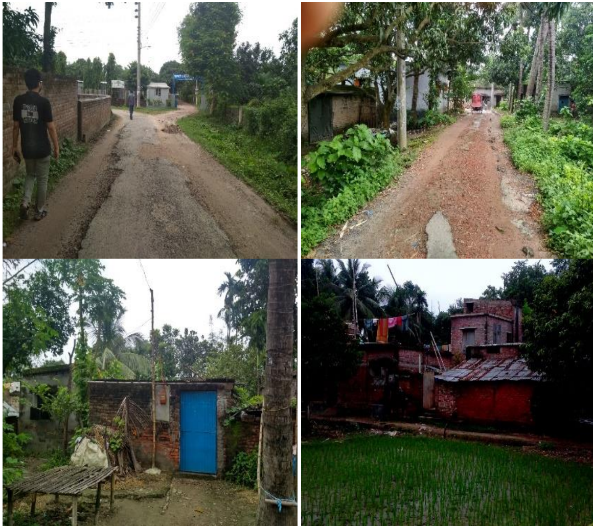
Fig. 2: Existing road and housing conditions.
