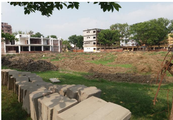
Fig. 3. Playground Fill up with Soil for Future Building Construction.
