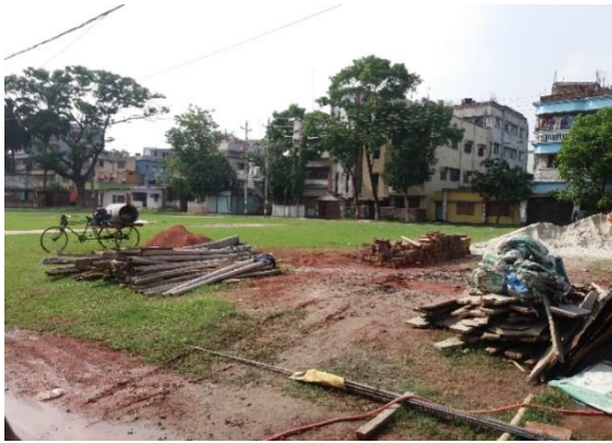
Fig. 2. Playground Filled with Construction Materials.
