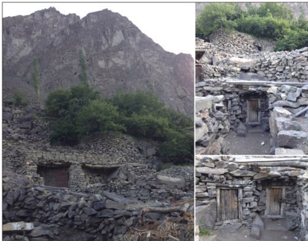
Fig. A3. Traditional storage facilities to deal with emergencies and extreme climatic conditions in Turtuk village, India. Source: Bayes Ahmed, fieldwork, July 2017.
